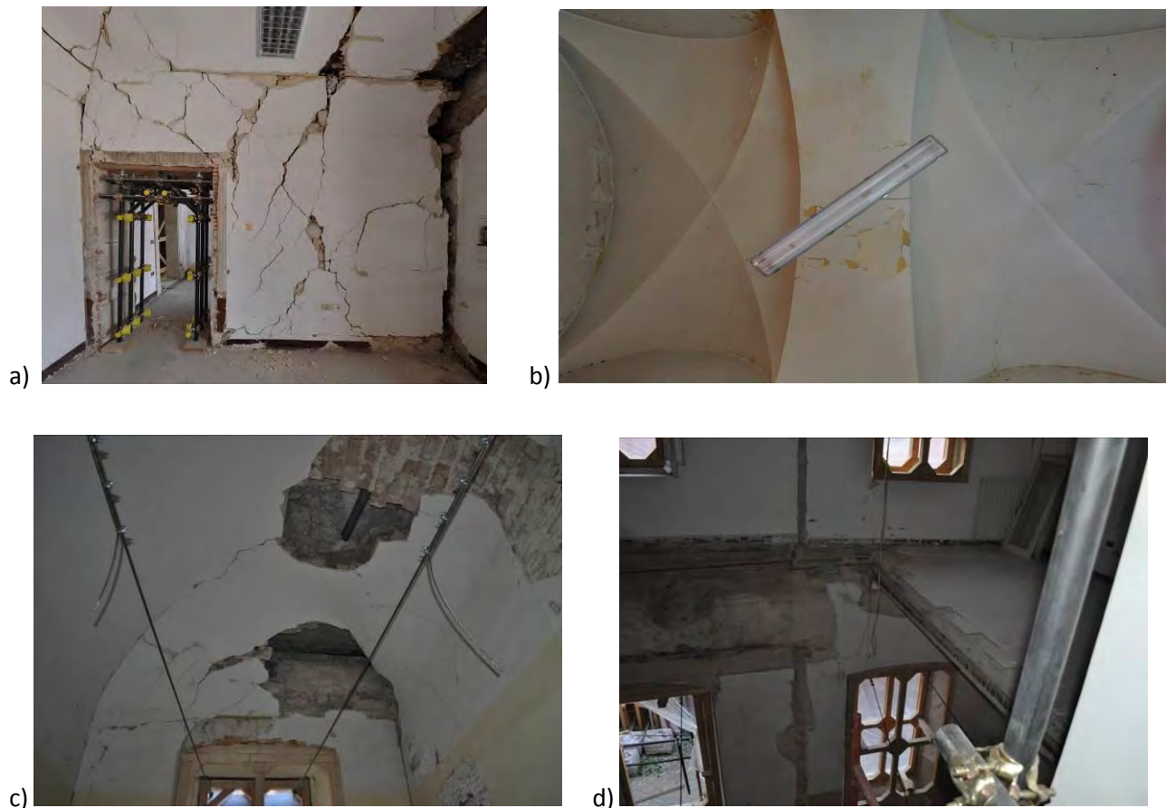
Fig. 4 – a) Diagonal cracks due to in plane action resulted in extended portions of the resisting walls: out of plane displacement have been recognized in few front walls of the building; b) typical geometry of cross vaults system; c) partial collapse of a trough vault; d) Part of a floor collapsed as consequence of the joist ends disengaged from the sustaining wall.
