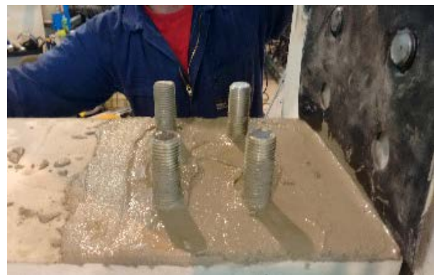
(b) Grout on beam surfaces
