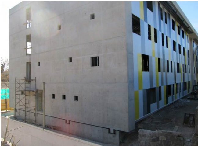
Figure 13: Shear wall west façade
