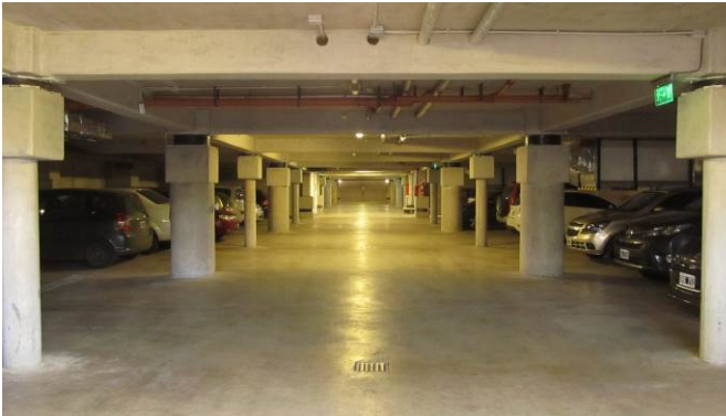
Figure 8: Isolators under the first floor
