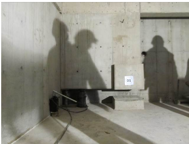
Figure 18: Core shear walls lifted as one unit
