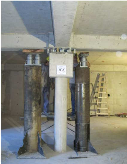
Figure 15: Temporary support
