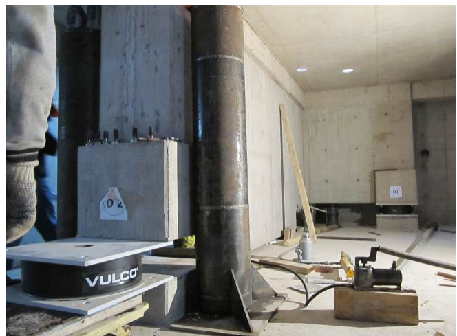
Figure 19: Base isolators location
