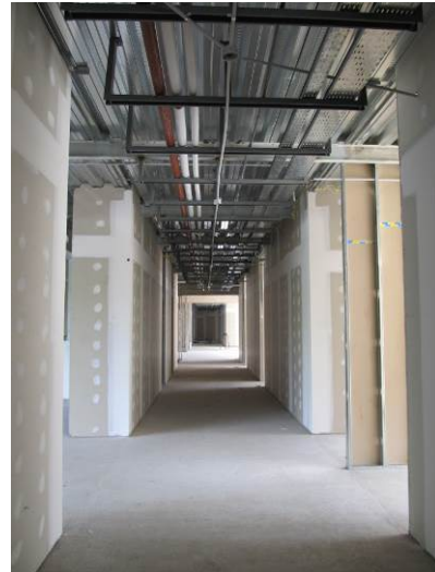
Figure 4: Internal partitions are plasterboard
