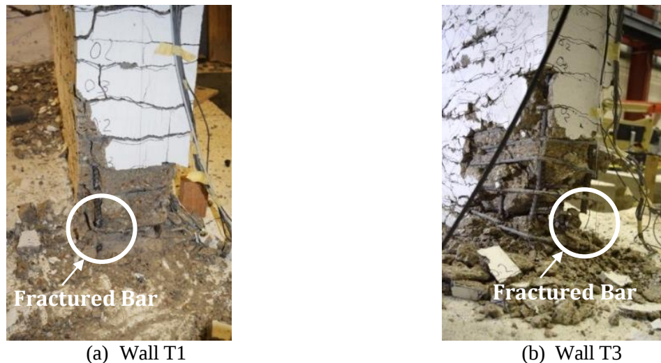
Fig. 8 – Bar fracture at confined stem during 4% drift cycle
