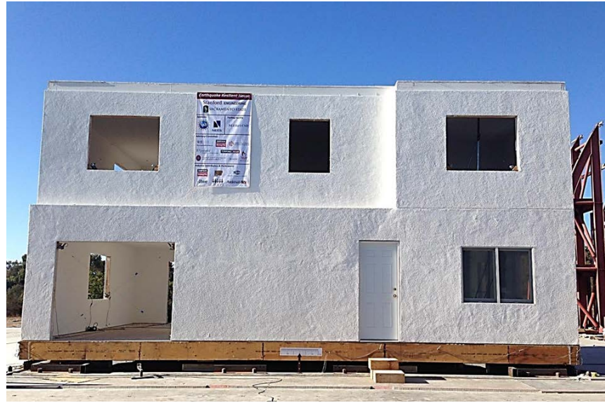
Fig. 4 - Full-scale sliding isolated house at NEES@UCSD.
