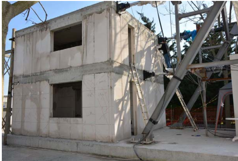
Fig. 12 – General view of the building after being tested to 2.0% drift ratio
