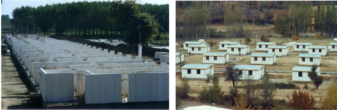
Fig. 2 – Post-earthquake housing units constructed with AAC reinforced panels [5]
