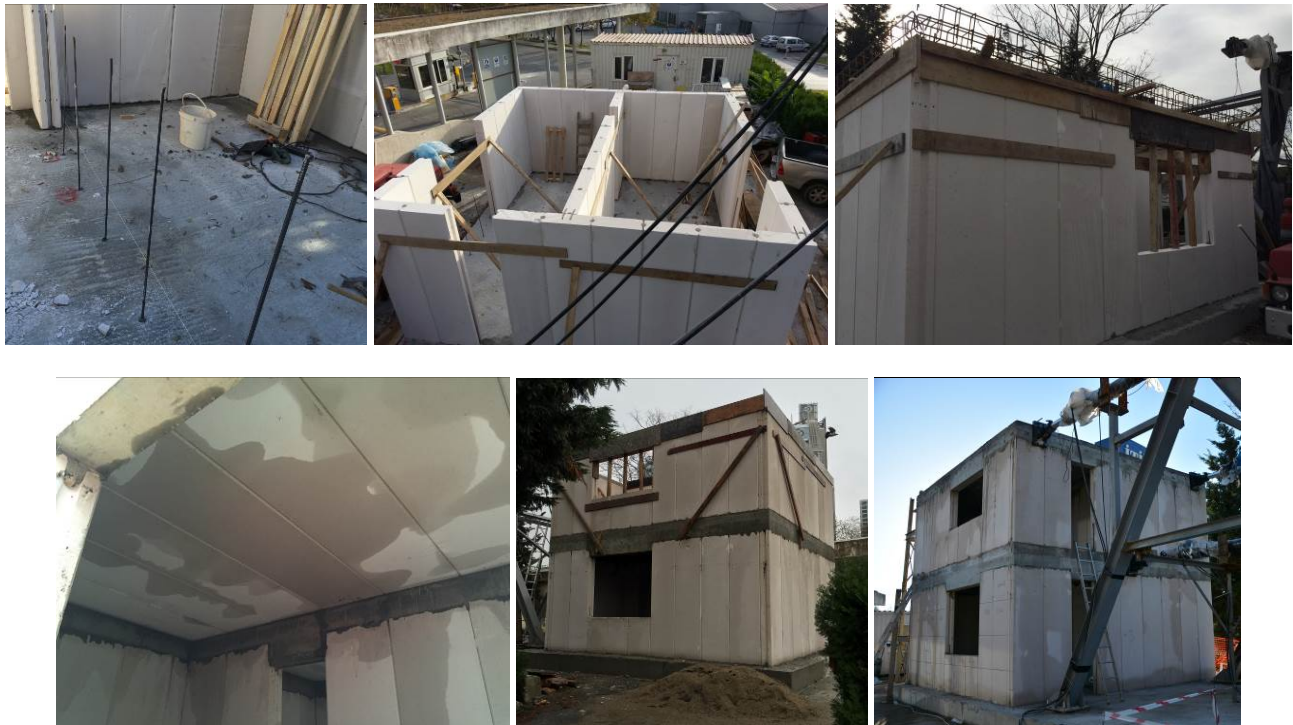
Fig. 6– Construction of the test building
