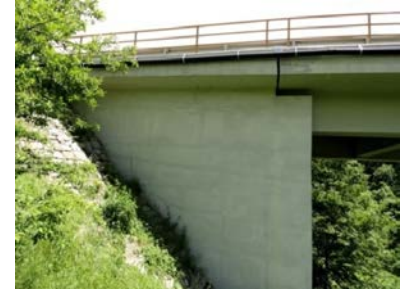
Fig. 4c. View of abutment of the selected prototype bridge
