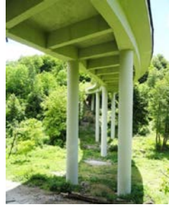
Fig. 4b. View of substructure of selected classical bridge structure
