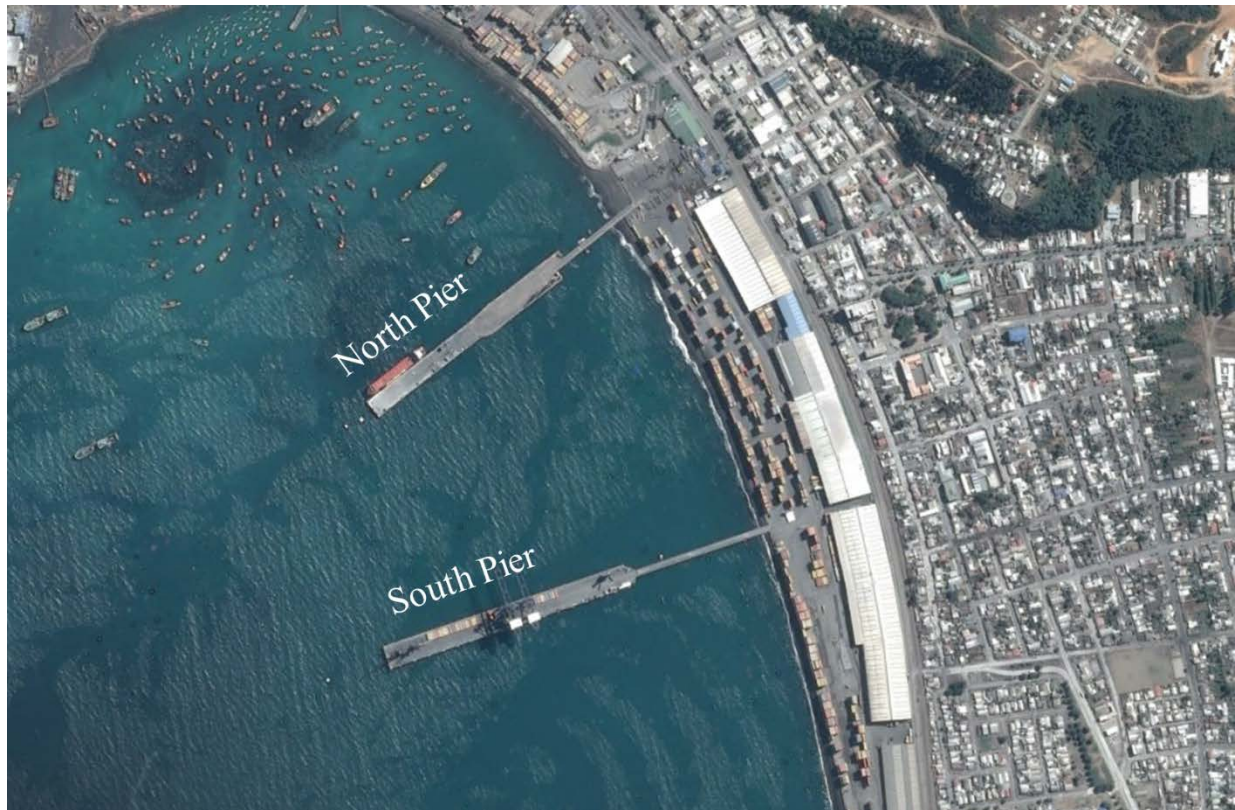
Figure 1 Piers damaged by lateral spreading
