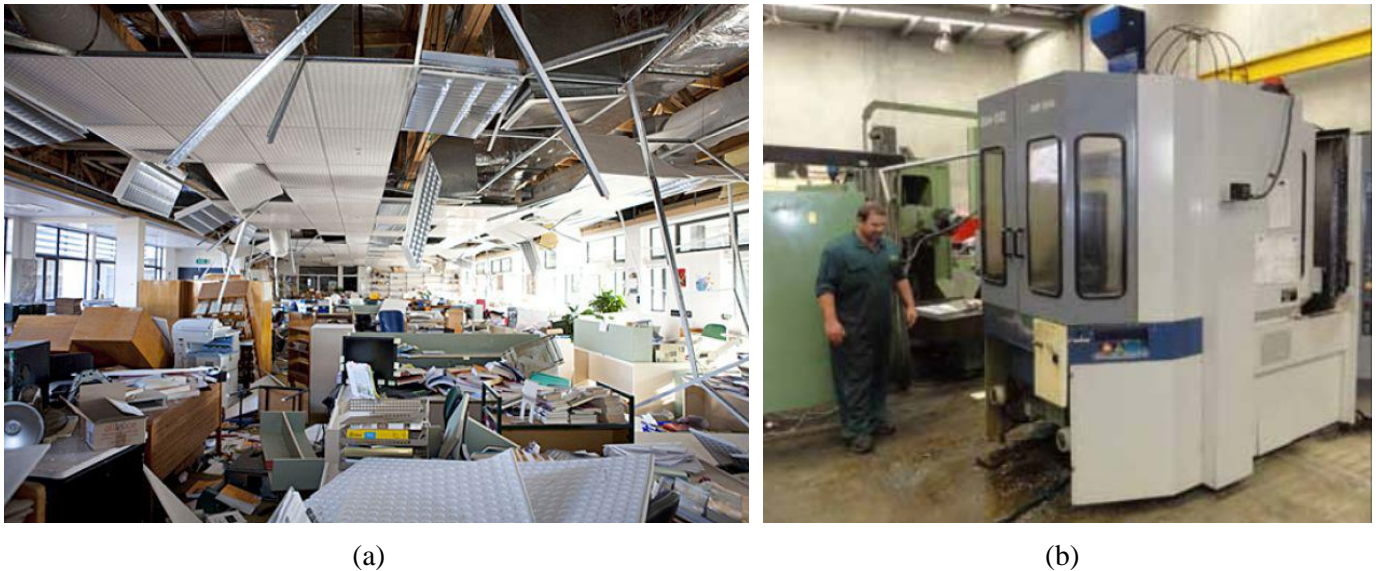
Fig. 1. Examples of damage to building contents: a) commercial environment (NIWA [20]), and b) displacement of heavy equipment in an industrial facility [19].
