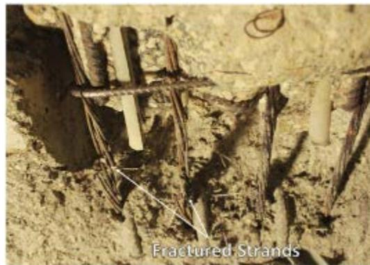
Fig. 8 – Fracture of Strands Providing Direction Tension Transfer
