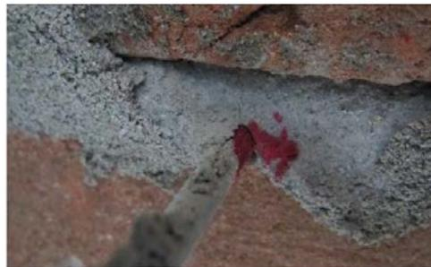
Fig. 20 and 21: Crack of mortar surface at brick tie connection location
