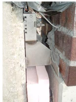
Fig. 4 – Supporting Construction
