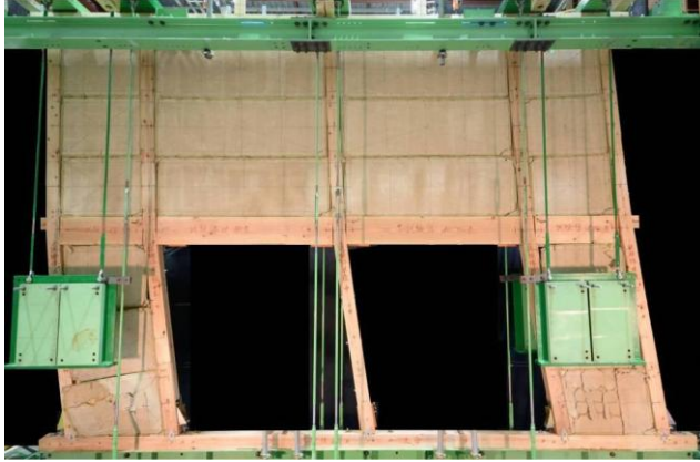
(a) Before collapse (First loop of R = 1/10\text{rad} )
