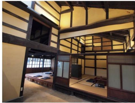
Fig. 1 – Example of structures with large hanging wall (Wakayama, Japan)
