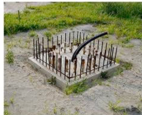
Fig. 4 - Moment-curvature relations for piles investigated Photo 1 - Damage to Illumination tower No. 54 [2]
