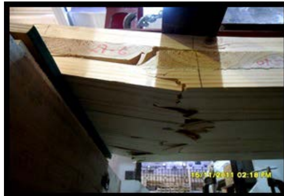
Figure 3 - Failure caused by bending
