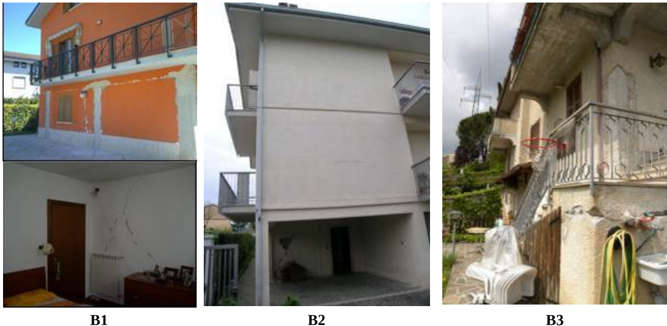
Fig. 1 – Overview of the case study buildings.
