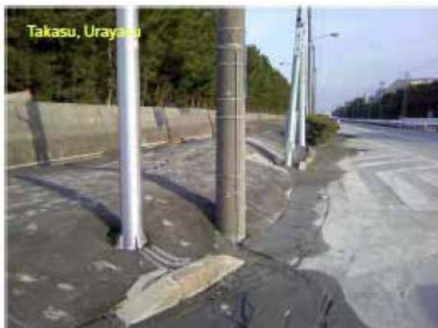
Fig. 2 Heaving of a footway in the Takasu district of Urayasu City
