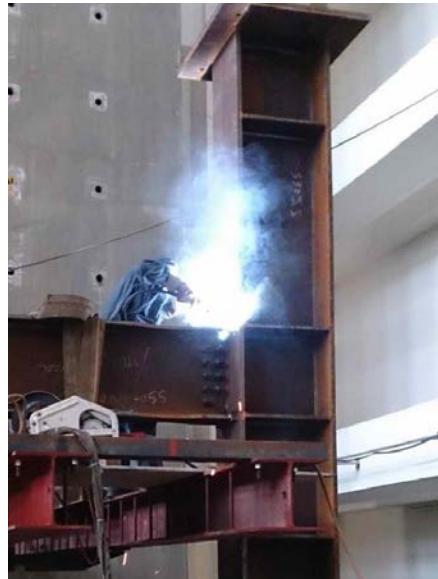
Fig. 3 – Completely joint penetration weld
