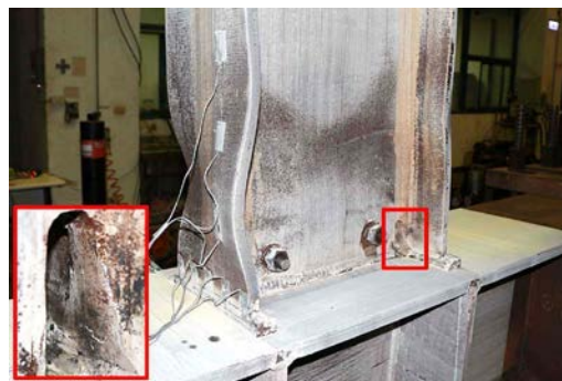
Fig. 8 – Local buckling and cracking at weld access hole of specimen WUF-W
