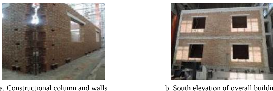
Fig. 2 – Construction of the masonry building
