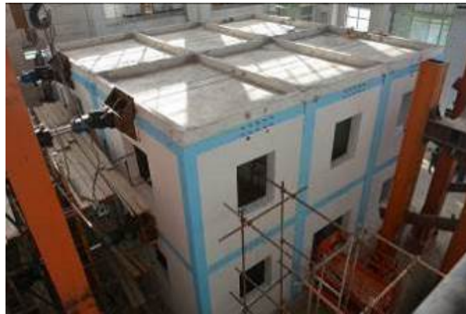
Fig. 8 – Repaired masonry building
