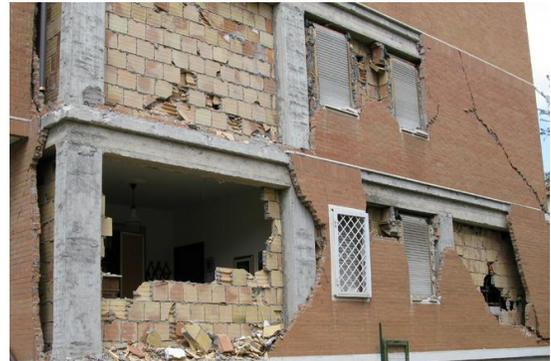
(b) damage suffered by a traditionally constructed infill wall during 2009 L'Aquila earthquake
