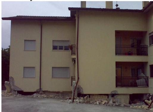
(c) building global collapse caused by the infill-frame interaction during 2009 L'Aquila earthquake
