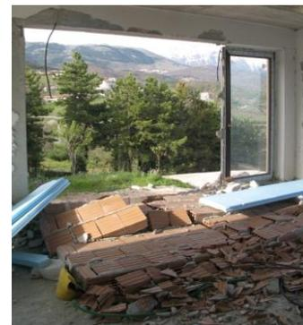
(d) out-of-plane infill overturning during 2009 L'Aquila earthquake
