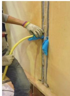
(e) mortar injection between sub-panel and vertical planks
