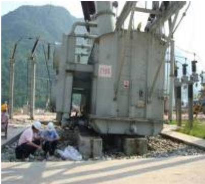
Fig.1 – Power Transformer falling platform
