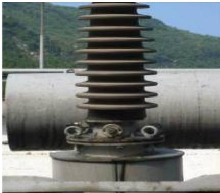
Fig.3 – Oil leakage at the bottom of casing
