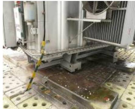
Fig.2 – Shift of power transformer
