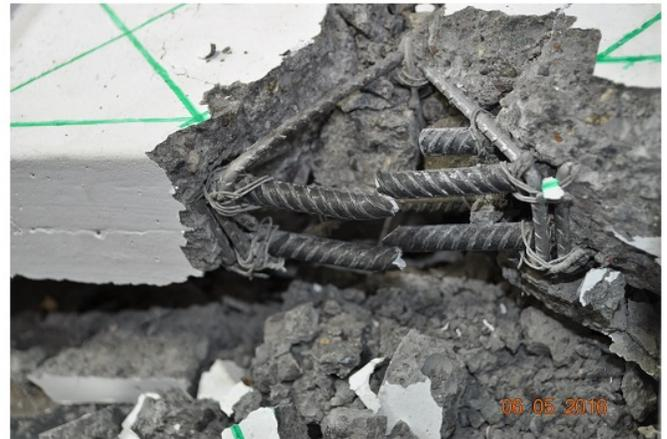
Figures 14: Inclined transverse hoops are not convenient for elements with low transverse reinforcement
