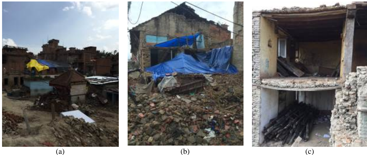
Fig. 2 – Overview of post-earthquake damage observed in Bungamati: (a) widespread damage to unreinforced masonry structures, (b) complete collapse of an example masonry structure, and (c) example flexible timber-diaphragm floor system.
