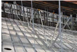
(b) Seismically designed ceiling with seismic coefficient of 1.1G (c) Seismically designed ceiling with seismic coefficient of 2.2G
