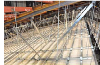
(b) Seismically designed ceiling with seismic coefficient of 1.1G (c) Seismically designed ceiling with seismic coefficient of 2.2G
