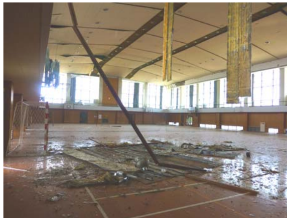
Photo 1 Collapse of Suspended Ceiling in Gymnasium during Kumamoto Earthquake
