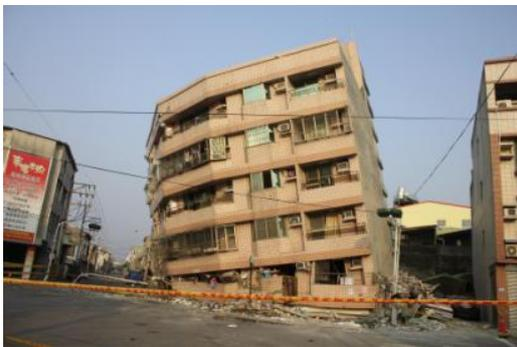
Fig. 8 – Buildings at the corner of an intersection collapsed in the 0206 Meinong earthquake owing to eccentric rotation
