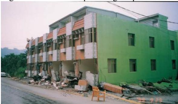
Fig. 1 – Collapse of the ground floor of a typical townhouse-type street house
