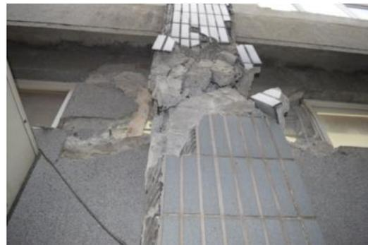
Fig. 9 – Shear failure of short columns in high windows
