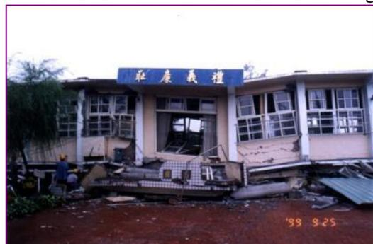
Fig. 2 – Collapse of the ground floor of a school building
