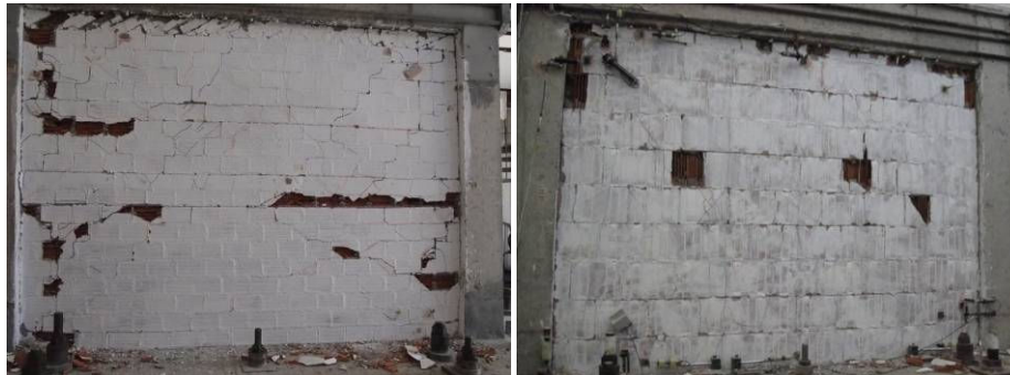
Fig. 10 – In-plane tests. Cracking of the CIS and INSYSTEM 2 specimens at maximum imposed drift.
