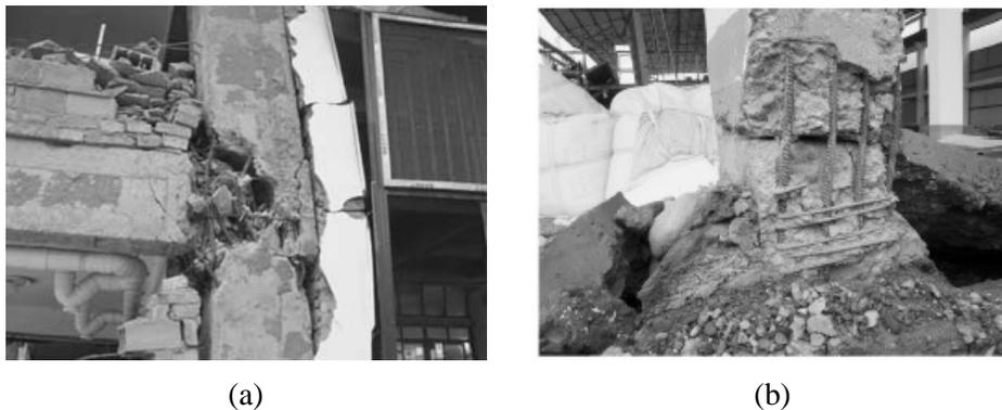
Fig. 1 – Damage of concrete frames after Wenchuan earthquake in 2008
