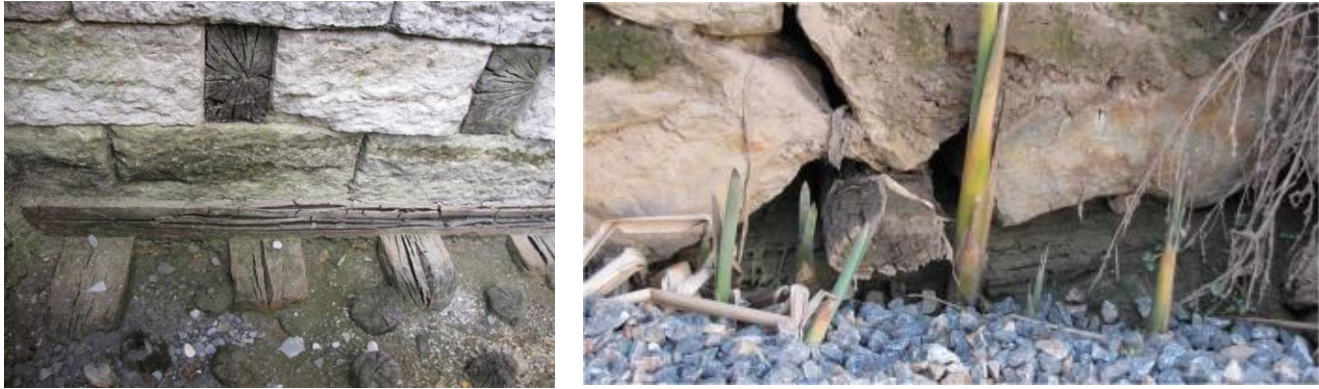
Figure 6. Wooden grillage of a Üsküdar and Sirkeci Byzantine chapels in Istanbul
