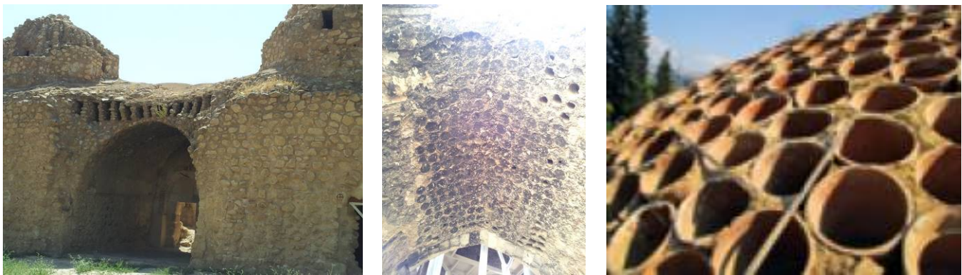
Figure 3. Reducing the weight of the vault or dome
