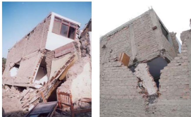
Fig. 1 – Masonry buildings that collapsed in 2007 Pisco earthquake [3].
