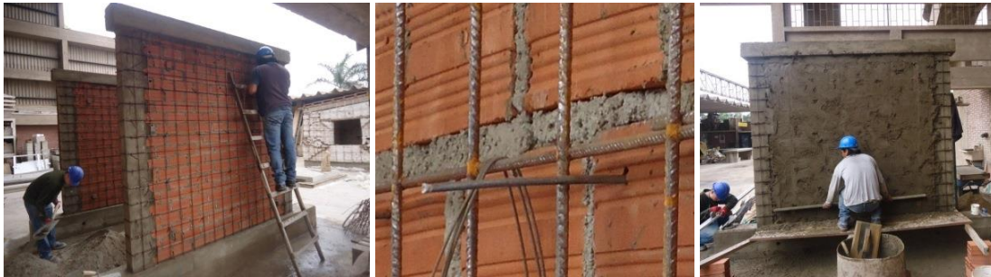
Fig. 7 – Placement of the welded wire mesh (left), connecting wires (center), mortar cover (right)
