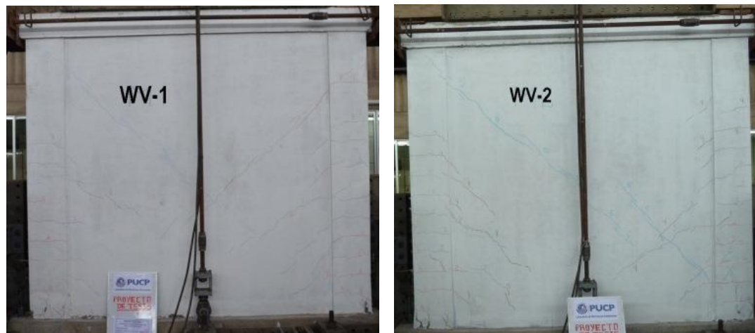
Fig. 9 – Wall WV-1 (left) and wall WV-2 (right), step 5.
