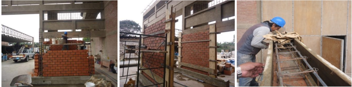
Fig. 6 – Construction of the masonry walls (left), tie-columns (center) and tie-beam (right)
