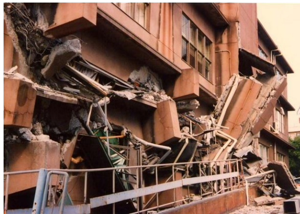
Fig. 1 Axial collapse (1995 Kobe Earthquake)
