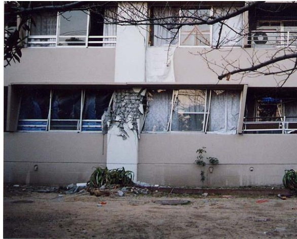
Fig. 2 Shear-damaged pattern with crushed core-concrete (1995 Kobe Earthquake)
