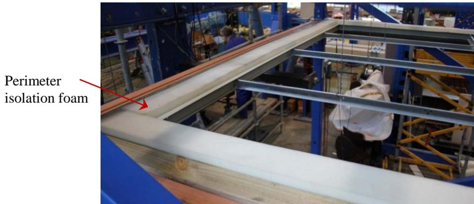
Figure 11 - Isolation foam placed in and filling the perimeter gap
