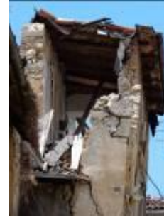
Fig. 11. Partial overturning of the external leaf of a perimeter wall of a masonry building in Sant'Eusanio Forconese
