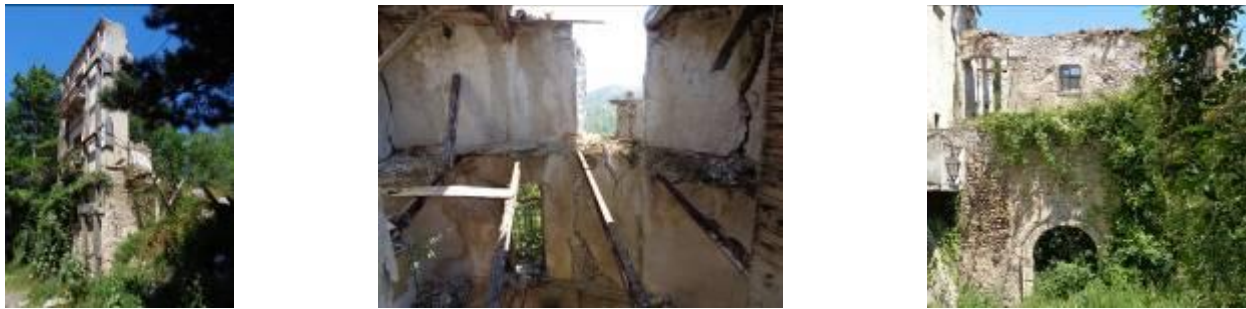
Fig. 6. The observed buildings' collapses in San Benedetto in Perillis
