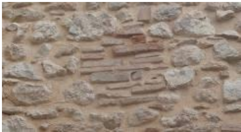
Fig. 4. Anti-seismic strengthening interventions observed in some of the studied minor historic centers: (a) Iron ties with different type of anchor plates and (b) buttresses observed in San Benedetto in Perillis; (c) “Scuci and Cuci” intervention in Bazzano and (d) Reinforced plaster in Castelvechio Subequo
