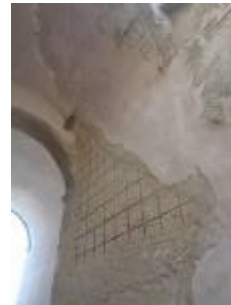
Fig. 4. Anti-seismic strengthening interventions observed in some of the studied minor historic centers: (a) Iron ties with different type of anchor plates and (b) buttresses observed in San Benedetto in Perillis; (c) “Scuci and Cuci” intervention in Bazzano and (d) Reinforced plaster in Castelvechio Subequo
