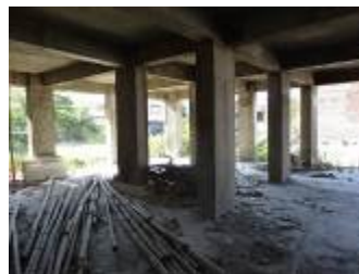
Fig. 5 – Rectangular shaped columns (KF)
