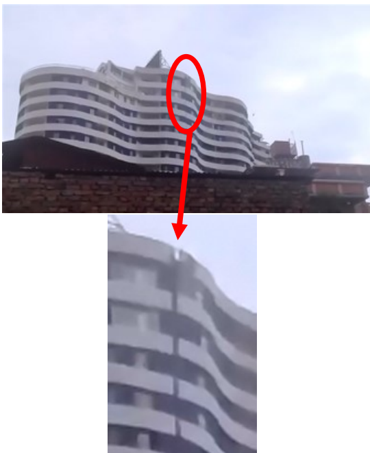
Fig. 14 – Building KE pounding behavior [2]
