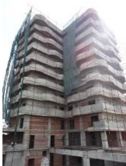
Fig. 3 – RC frame with infill brick Wall (KG)
