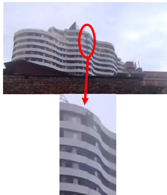
Fig. 14 – Building KE pounding behavior [2]
