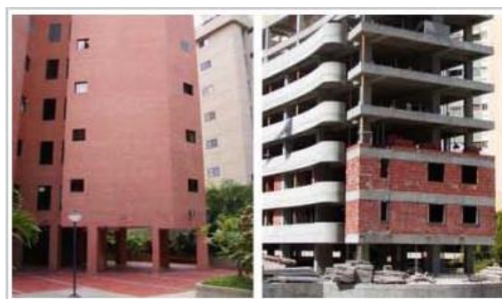
Fig. 1 - Example of buildings, structured with reinforced concrete frames and infill masonry walls, where the first story is likely to develop a soft story ( www.ingcivil.org )
