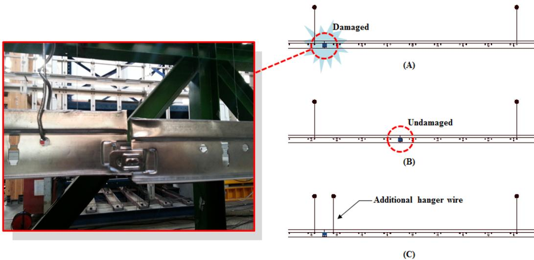
Fig. 19 –Damage to the connection joint of the main runner
