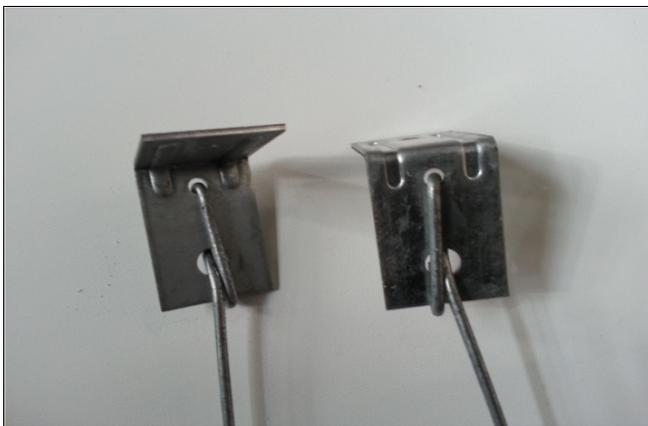
Fig. 8 – Hanger wires and connection devices
