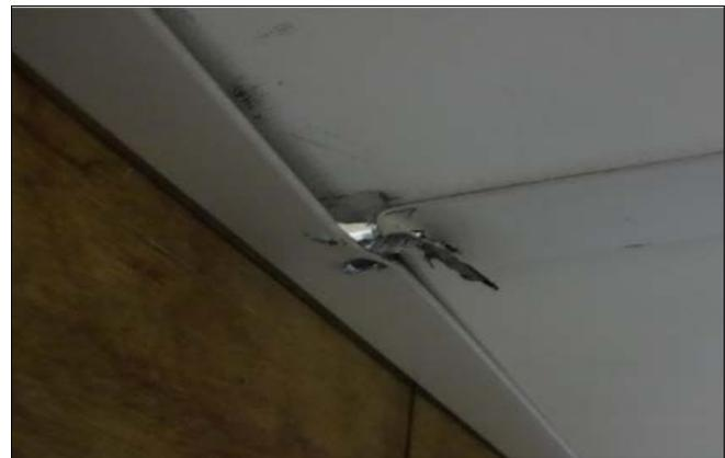
Fig. 16 – Failure of perimeter connection
