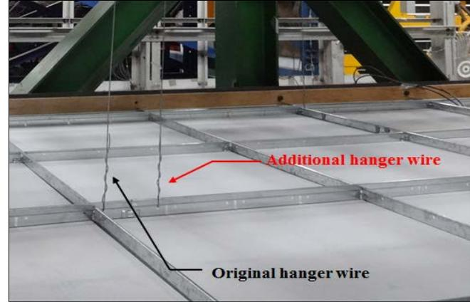
Fig. 12 – Installation of the additional hanger wire
