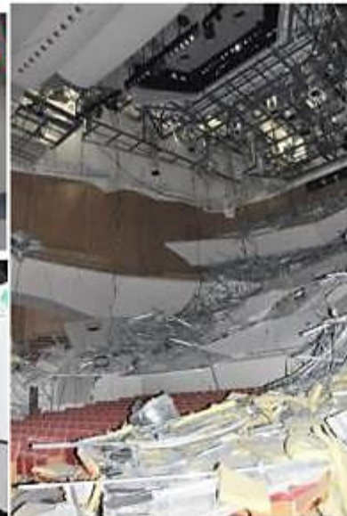
(a) Lab. (Clean room) (b) Sport Entertainment (c) Concert hall Photos.3 Damage examples of ceilings w/o clearance in the Great East Japan Earthquake
