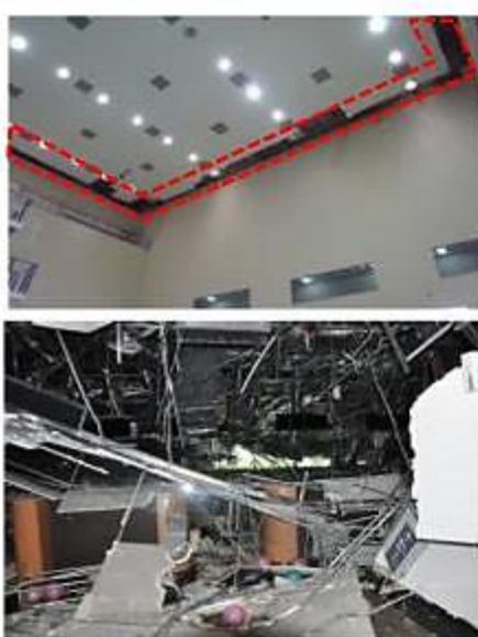
(a) Lab. (Clean room) (b) Sport Entertainment (c) Concert hall Photos.3 Damage examples of ceilings w/o clearance in the Great East Japan Earthquake
