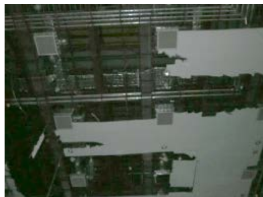
Photo.6 Ceiling fall in the target building
