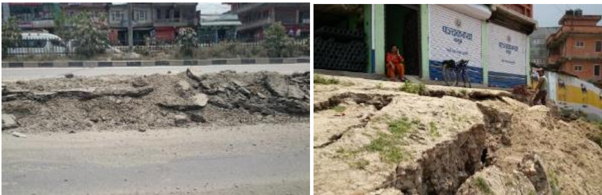
Fig. 11 – Ground deformation with vertical and horizontal offsets of approximately 2 m and 0.5 m respectively observed in Lokanthali region
