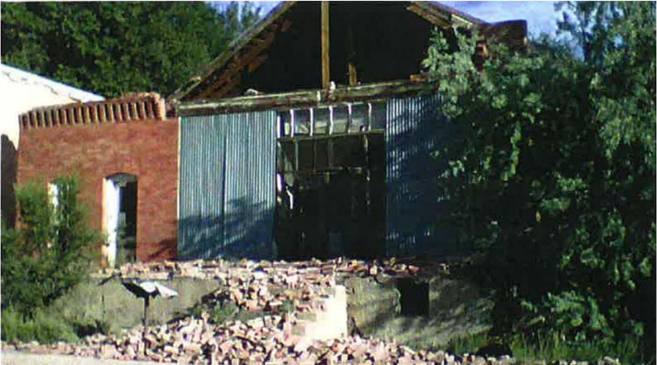
Fig. 2 – Damage to brick façade in Trinidad, Colorado due to 2011 earthquake.
