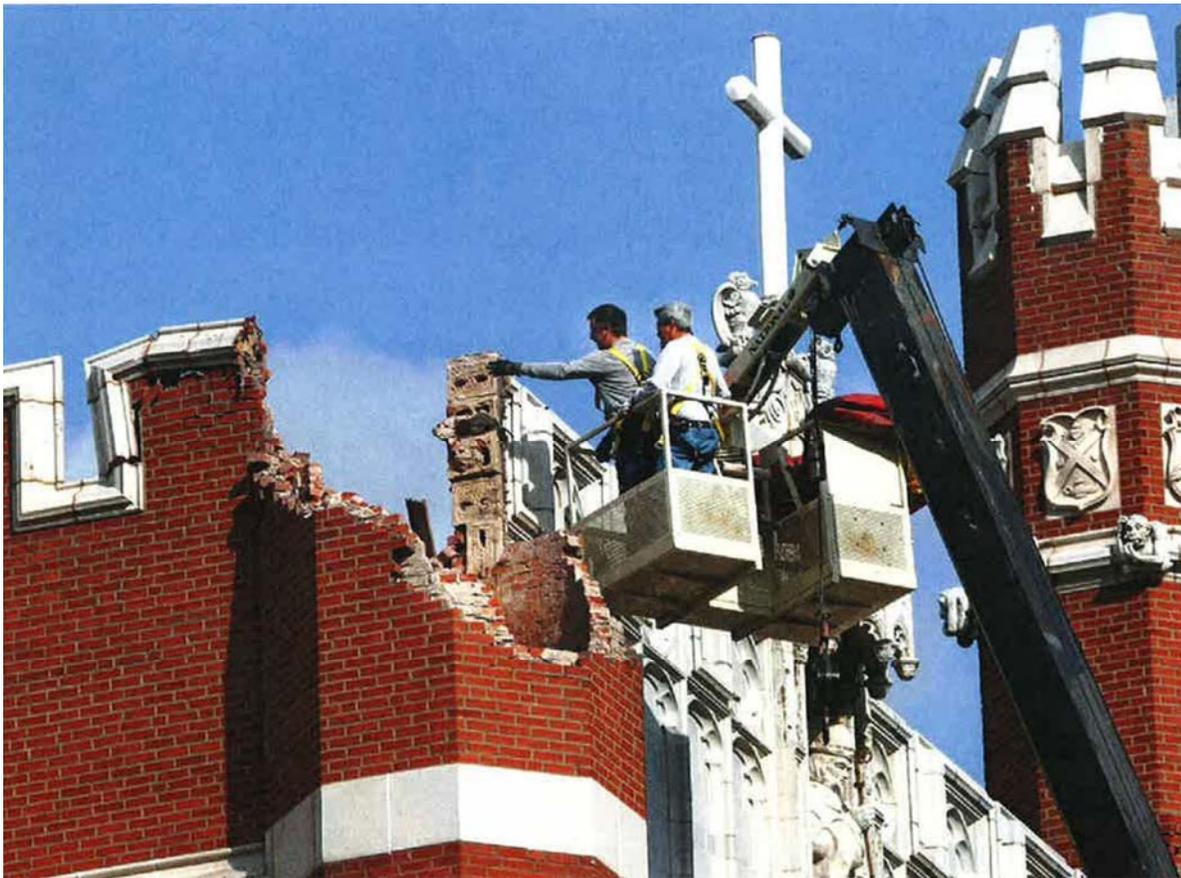
Fig. 1 – Damaged spire at St. Gregory’s University in Shawnee, Oklahoma due to the 2011 Prague earthquake.
