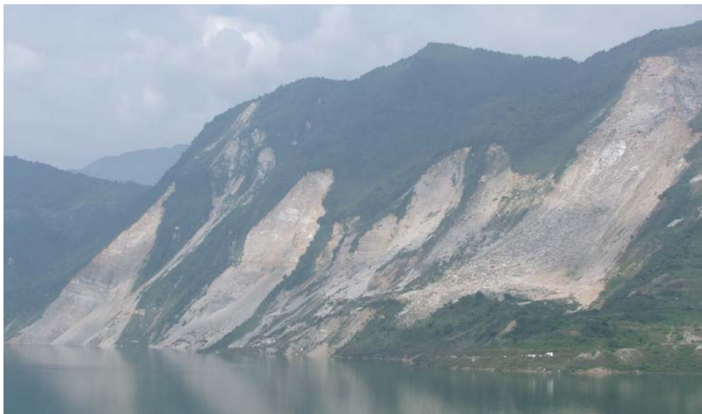
Fig. 1. Rockfalls in the Zipingpu reservoir area caused by the May 12, 2008 Wenchuan earthquake in China (photo taken from Zipingpu dam crest when reservoir was full, April 2009)
