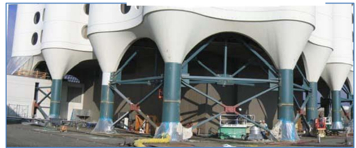
Fig.- 8 Saint Joseph Hospital, Patient Towers, Seattle, 40' Soft Story, Retrofitted with X-Brace PFDs.[15]
