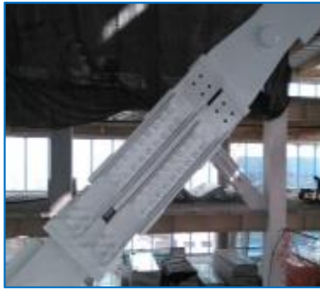
Fig.-18. PFD Assembly-3 in diagonal brace spanning over 2 floors.
