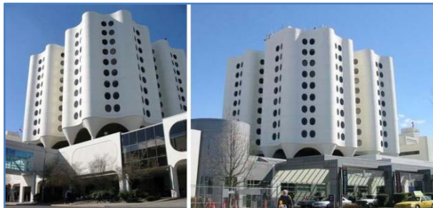
Fig.- 8 Saint Joseph Hospital, Patient Towers, Seattle, 40' Soft Story, Retrofitted with X-Brace PFDs.[15]
