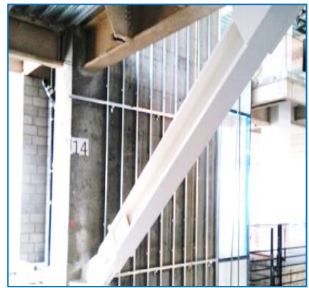
Fig.-19. This brace is continuation of brace in Fig. 18, serves 2 floors.
