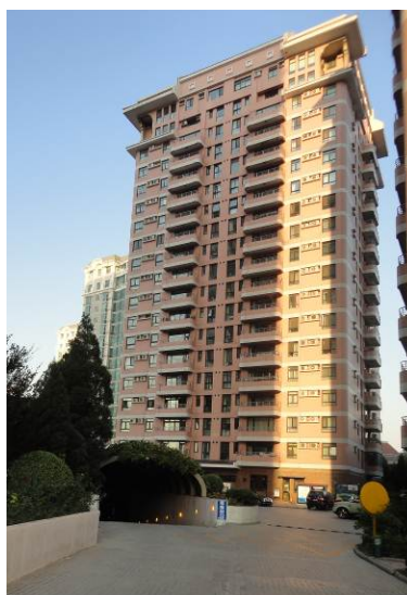
Fig. 1 – General view of the 20-floor concrete shear wall building
