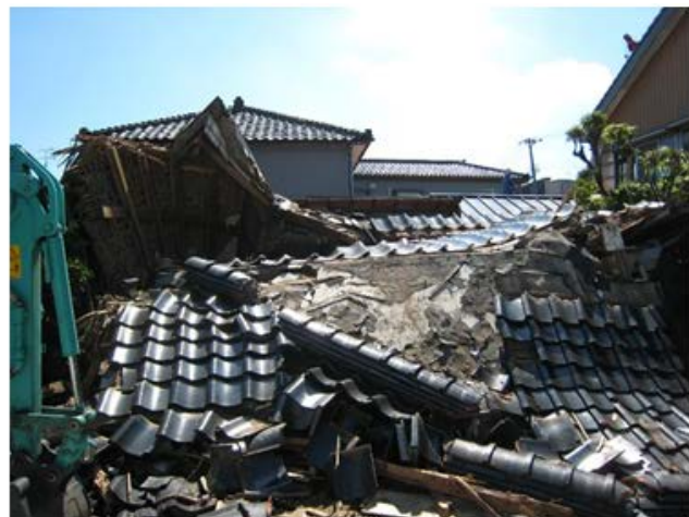
Fig. 2-3(2). Examples of photos of a critically damaged wooden house and estimated values on volumetric loss
