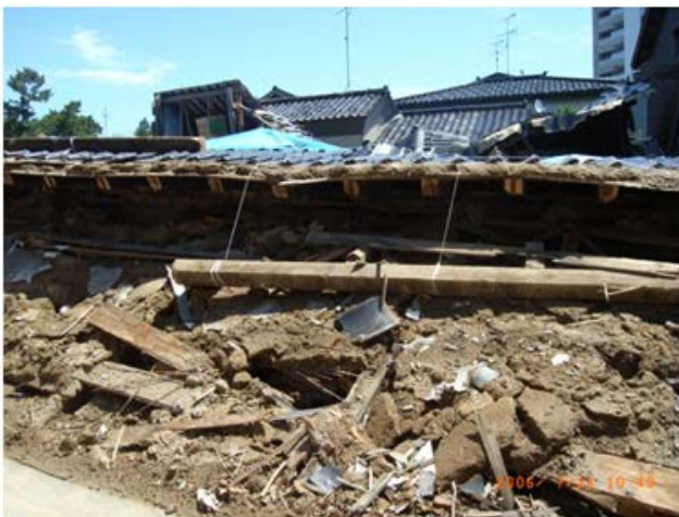
Fig. 2-3(2). Examples of photos of a critically damaged wooden house and estimated values on volumetric loss
