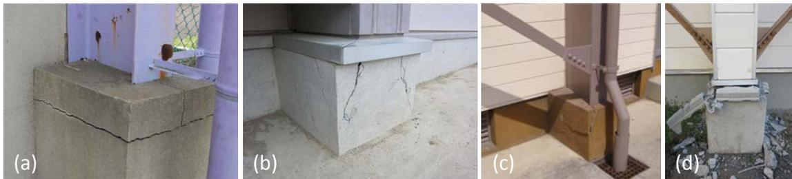
Fig. 1 – Damage to concrete foundation of exposed column base in the 2011 Tohoku earthquake [2]
