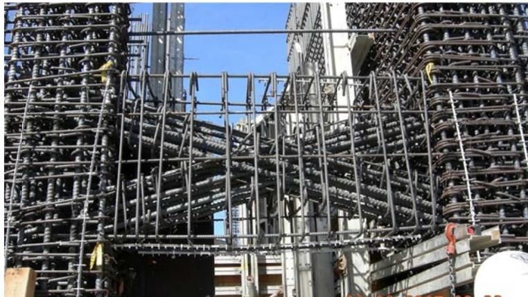
Fig. 1 – Reinforcement congestion in a diagonally reinforced coupling beam (courtesy of Rémy Lequesne)
