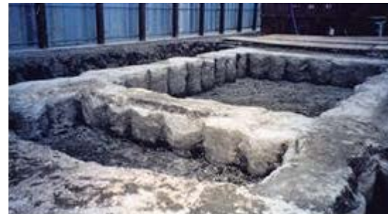
Phot.2 Grid-wall soil improvement.
