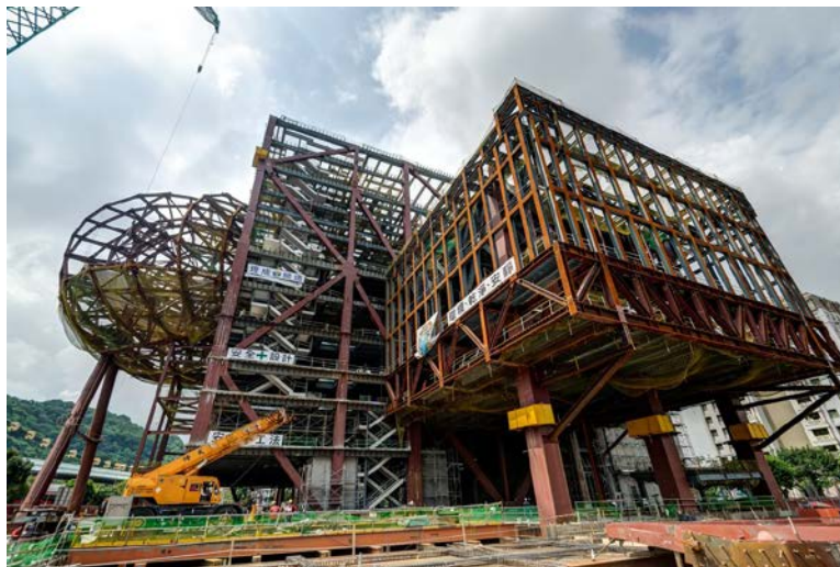
Figure 14. Construction photo taken at the TPAC site in March 2014 (by OMA)
