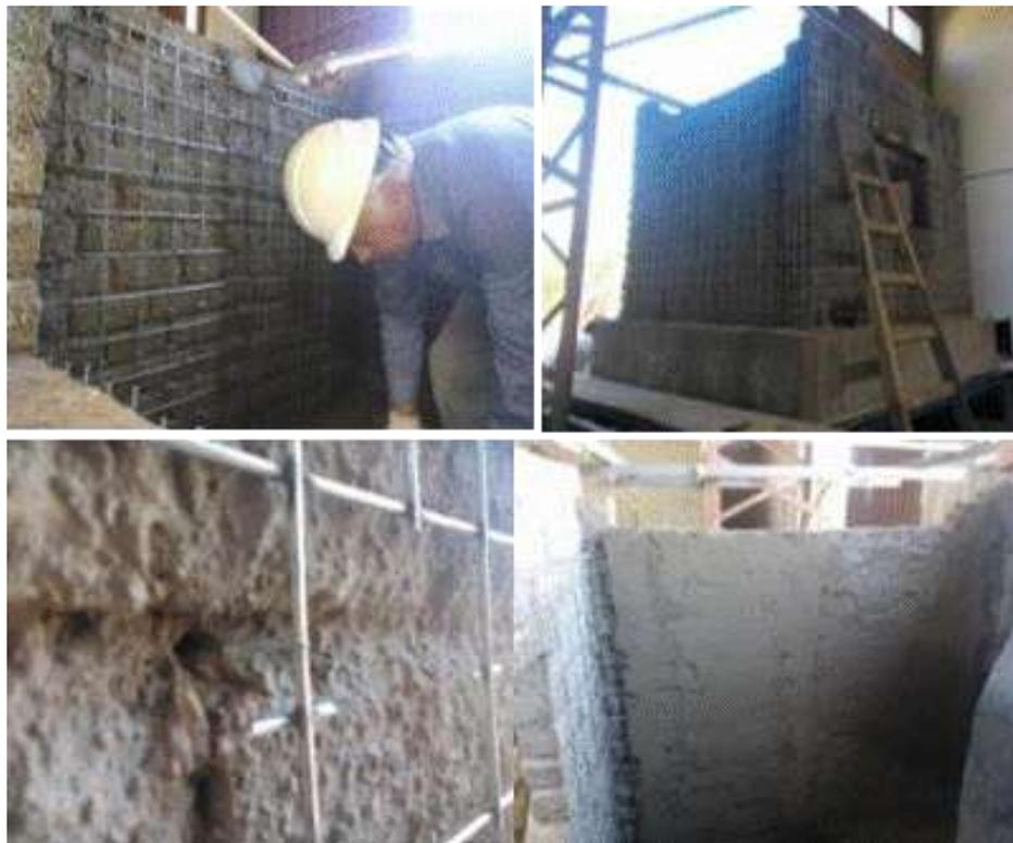
Fig. 9- Positioning of the steel mesh and plaster covering application.
