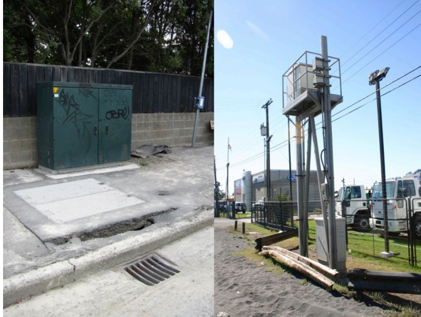
Fig. 5 – Roadside cabinet on the left and pole mounted cabinet on the right
