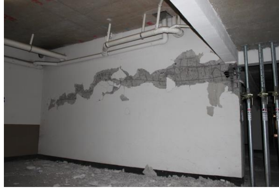
Fig. 1 – Sample image of reinforced concrete shear wall damage in the 2010 Chile earthquake [11-13]
