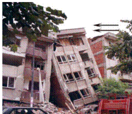
Fig. 2- One of the adjacent buildings pounding to another building and changing its direction during Marmara earthquake in Turkey [7]
