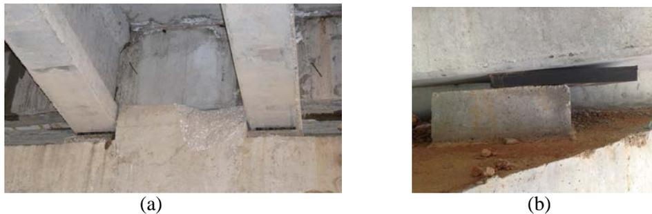
Figure 1. (a) Shear key damage during an earthquake (b) walkout during service
